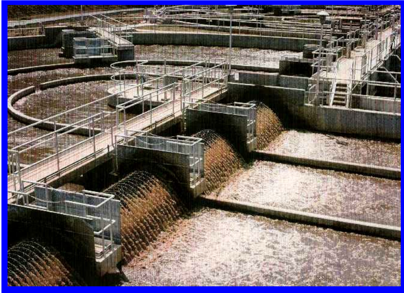
Horizontal disk aerators in action with little spray or aerosol formation
