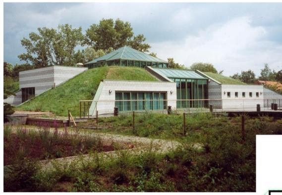
completeley covered full odour control noise control + unobtrusive : - can be built underground - camouflated
