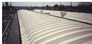
Our fixed VOC containment cover systems reduce the risk of explosions by using an inert gas, such as nitrogen, instead of air.
