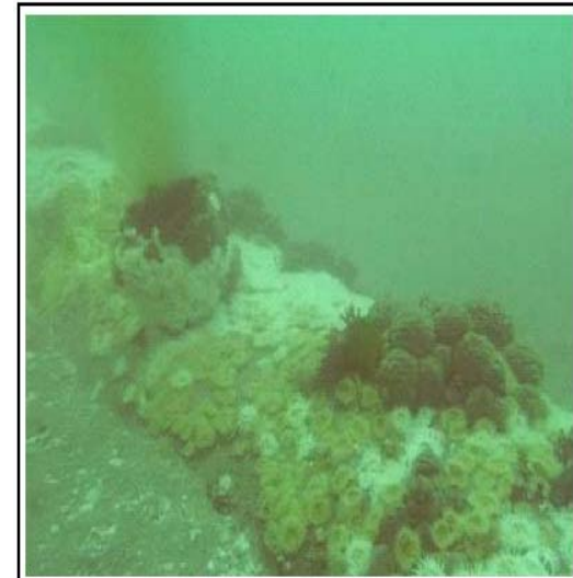
(Underwater) Diffuser Section of Outfall on Sea Floor
