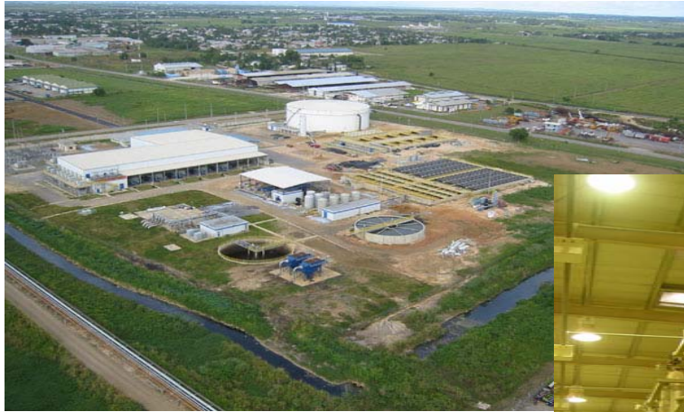
Seawater - RO & Thermal
