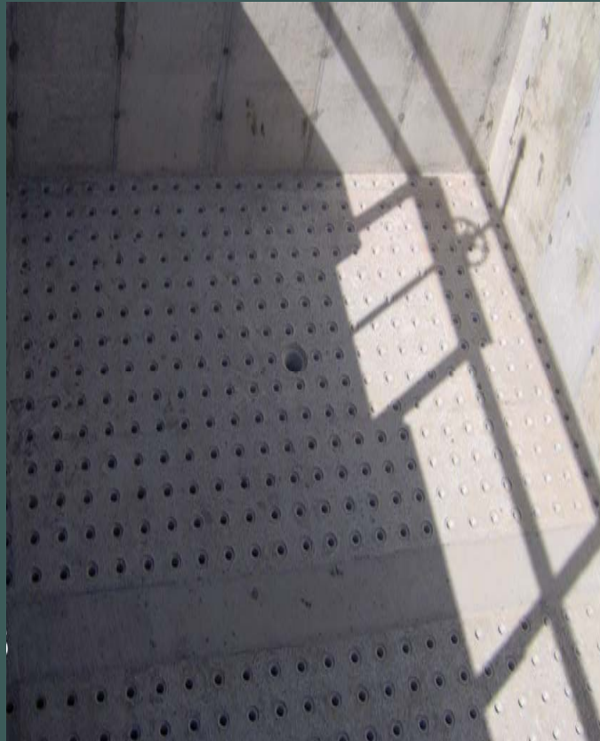
Biostyr Media Retention Platform
